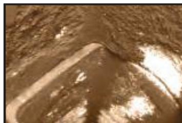
Actual photo of spalled flue tile
